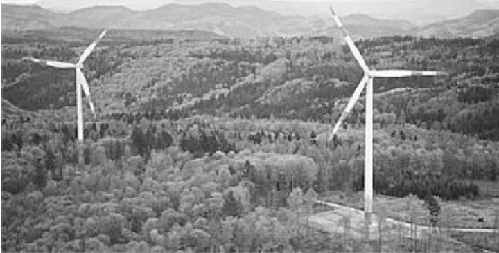
2 NORDEX 80 near Lahr (GER), height 120m, 2,5 MW
